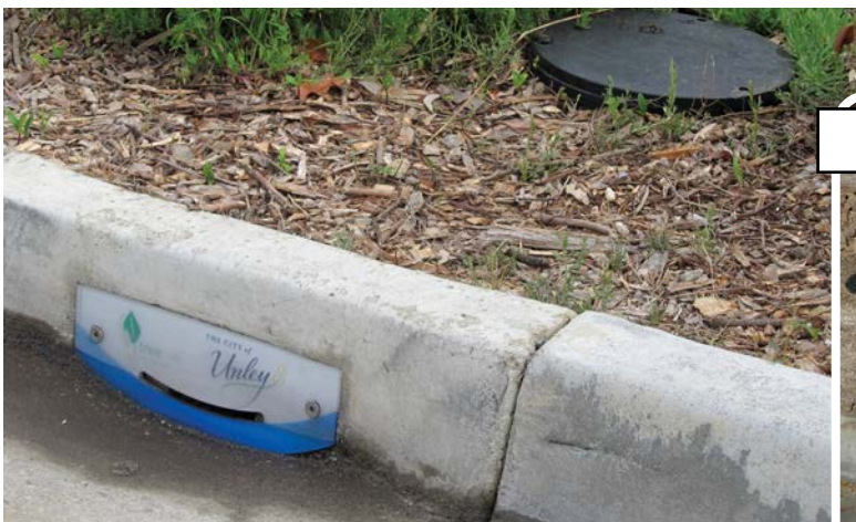
TreeNet inlets capture stormwater from water runoff and utilise the water to support tree growth.
