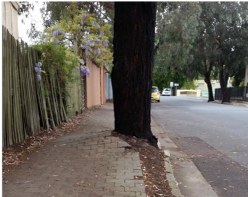
Figure 3.10: Footpath Damage on Nichols Street
