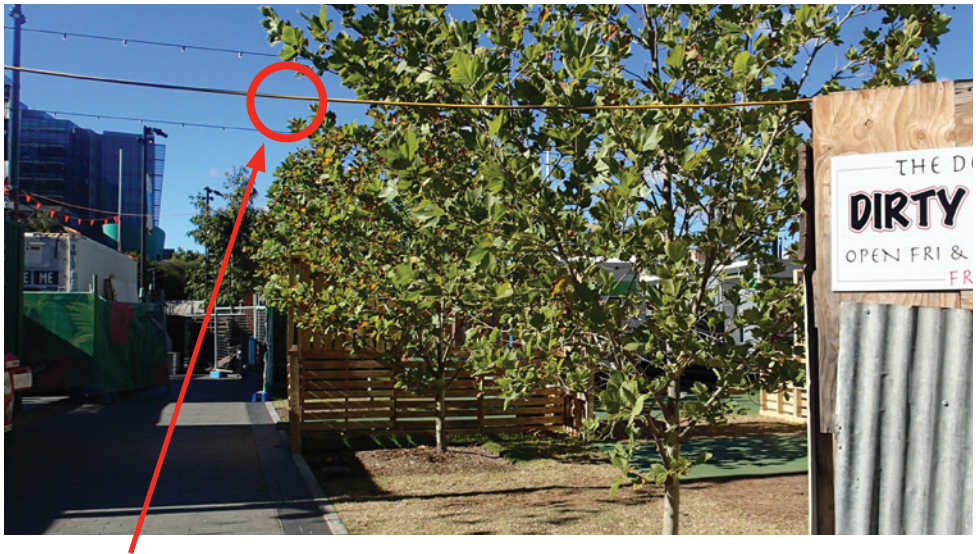
The cable in the foreground is not installed correctly, as it is too low, has no secondary support, and is not flagged.
